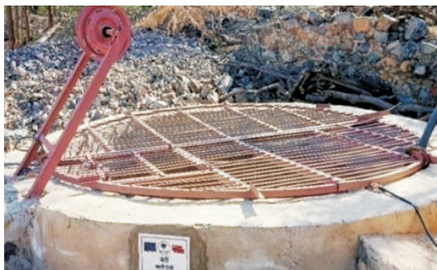
Renovation of open well at NICRA village
